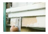
APPLYING MINERAL PAINT All new rendered surfaces should be properly dry before applying lime paint. Apply with a good quality long haired brush in short strokes. Do not overload the brush, using only the bottom third of the bristles. Uneven application will result in uneven colouring. Stir paint regularly during application. Generally, two coats are sufficient. Wait 6 to 12 hours between coats.
