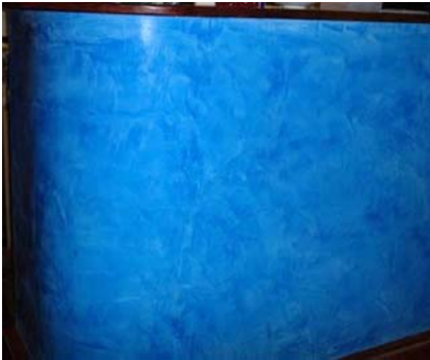
A marmorino on plasterboard + Decofond+ Decoliss (no intermediate coat)
