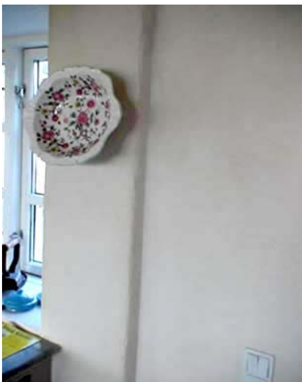
Chase area, finished
