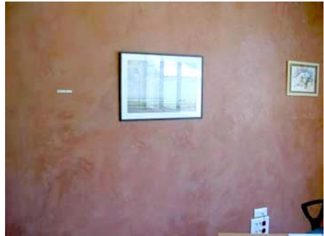
Polished stucco on Decofond.
