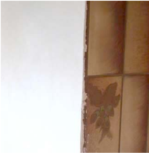
Plastering directly on tiles
